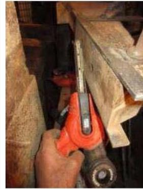
measured up and made sure they were parallel and square again. The space and access was so restricted that I couldn't get in with the meat cleaver, so I resorted to the power file only, working with a sweeping action. It only has a pad behind a small area of the narrow sanding belt.
