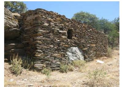
The oil mill with an old flat stone in the wall. One can see the wall built against the cliff to enlarge the cave.
