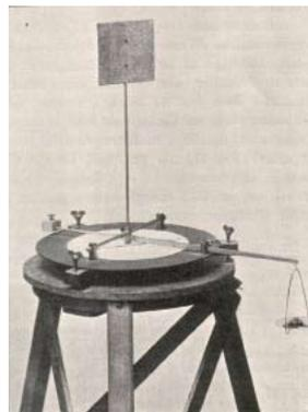
La Cour made measurements on a plane, a curved and a bent wing profile. The bent profile gave the best results, and the measurements were presented in his research report, Forsøgs-møllen I and II, year 1900.
